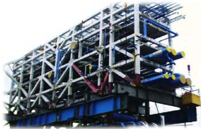
Steel structure for Åsgaard B – (Client: Kværner)
