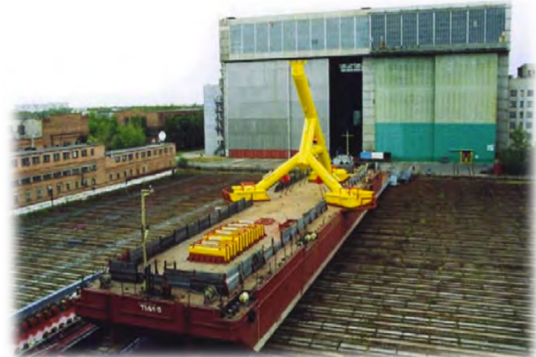
Tide mill structure - delivered to ABB
